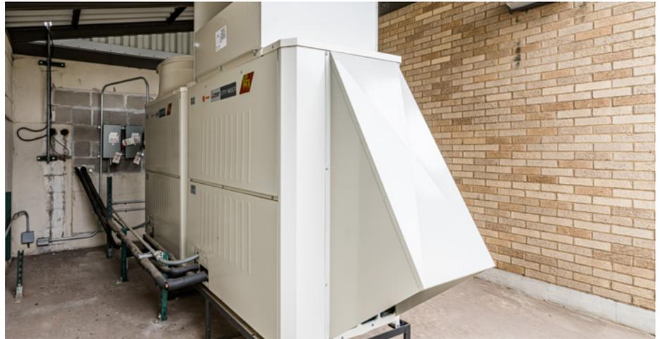
air. 12 Smart MEs and one AE-200A Centralized Controller were specified for system management. Each tie in to Minnesota’s Power’s building automation system at their Duluth headquarters location, streamlining efficiency and comfort control.
