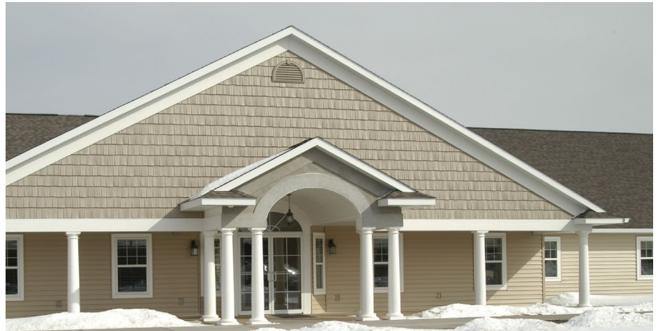
The Mitsubishi Electric VRF zoning system installed at the Brentwood assisted living facility provides individual and simultaneous cooling and heating to 29 units, the kitchen and a chapel.
